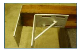
**Step 5:**Position inside corner (H-IC) making sure that it is square and tighten the bolt enough to keep brackets from moving.
