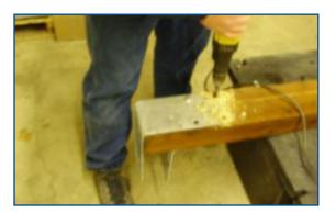
Drill and install remainder of carriage bolts, as shown.
