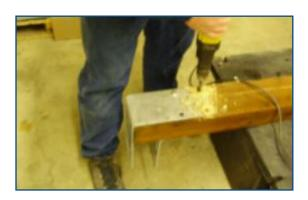
Drill and install remainder of carriage bolts, as shown.
