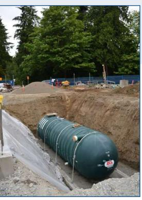
These large fibreglass tanks are commonly used for toilet and urinal flushing, process water in manufacturing facilities, heating & cooling applications and irrigation along with controlling stormwater runoff. They come in a wide variety of sizes, shapes and configurations and can be fitted with a number of different accessory packages. Just call BARR with your specific requirements and we'll be happy to find the best solution for your needs.
