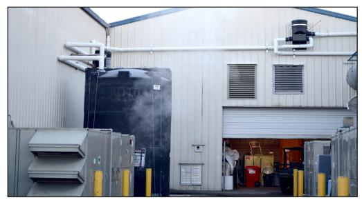
We worked with Abbotsford Water & Sewer Services to create an 8,000 USG ASTM rated poly tank system with engineered seismic tie-downs. This custom rainwater system collects from 48,000 sq. ft. of roof area to collect up to 1.6 million US gallons per year to flush over 30 bathroom fixtures. It was designed to meet the demands of a tradeshow day which can commonly use up to 8,000 US gallons.
