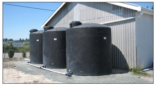
AW 9,000 USG system comprised of 3 tanks that collects from 5000 sq. ft. roof and supplies water for filling mobile equipment and washing equipment.
