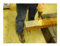
Drill and install remainder of carriage bolts, as shown.
