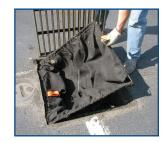
**To remove:** Simply lift the grate, grab the handle, and pull out the insert.
