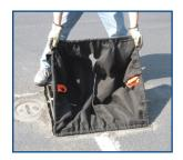
**To install:** Remove grate and adjust wire frame to fit in recess.
