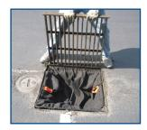
Place insert into recess and frame into corners. Replace the metal grate.
