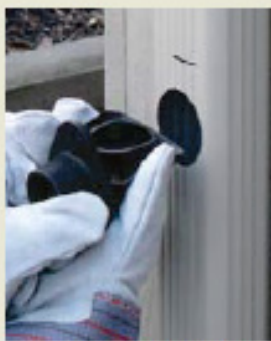
Insert FlexiFit™ diverter
