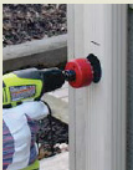
Drill hole in downspout
